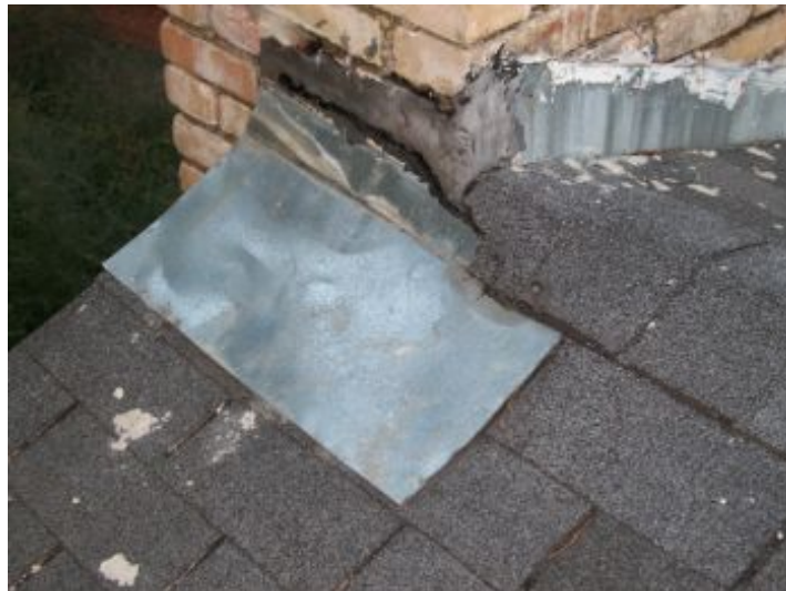
Evidence of repair around the chimney.
